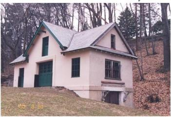
In May 2001, the east gatehouse was renovated. The floors had to be jacked up, the wood replaced, and new tile laid. The walls were sheet rocked, primed, and painted, and new wiring and receptacles installed. The total cost of \$1,250. was paid by the Comologuoy Trust.
